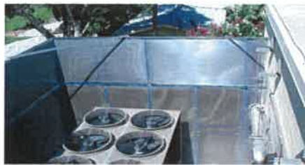
Panels prevented moving chillers
