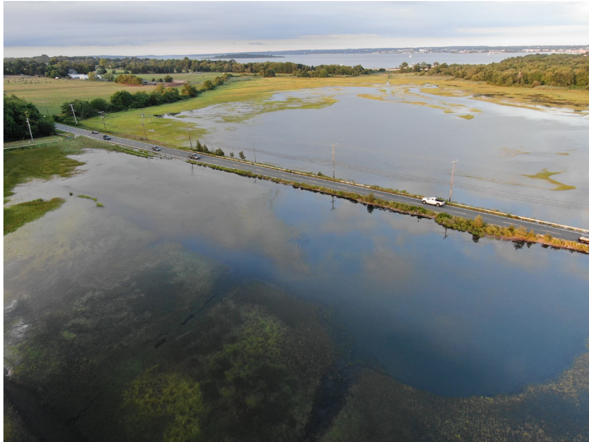
Existing Round Swamp Bridge #289
