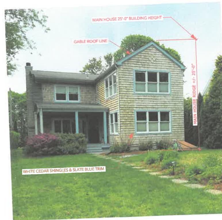
REAR ELEVATION OF MAIN HOUSE
