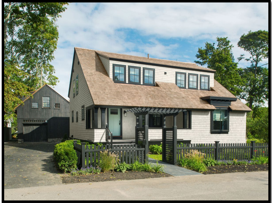
Source: This Old House (URL: https://www.thisoldhouse.com/jamestown-net-zero-house )
