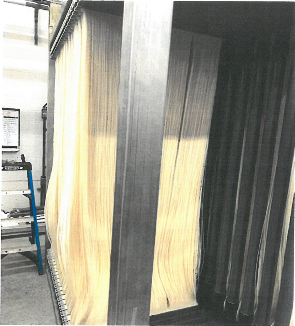
New membranes installed.
