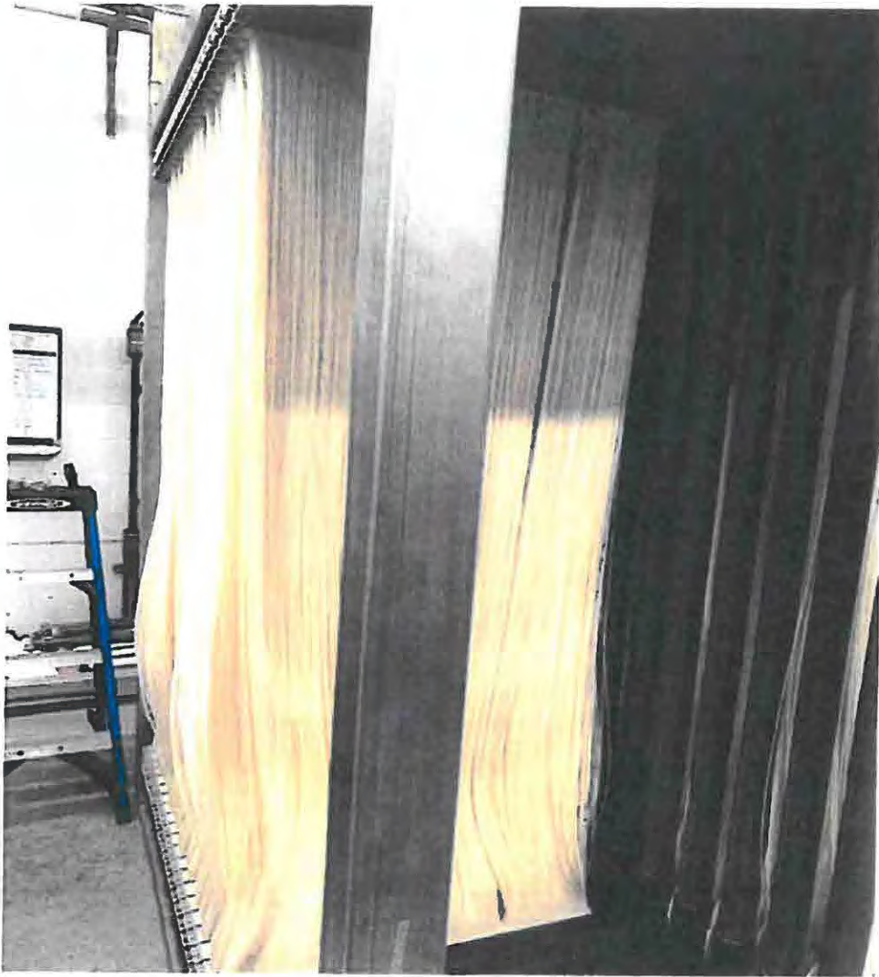
New membranes installed.
