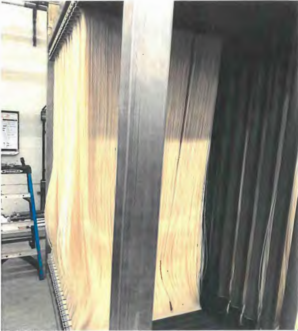
New membranes installed.
