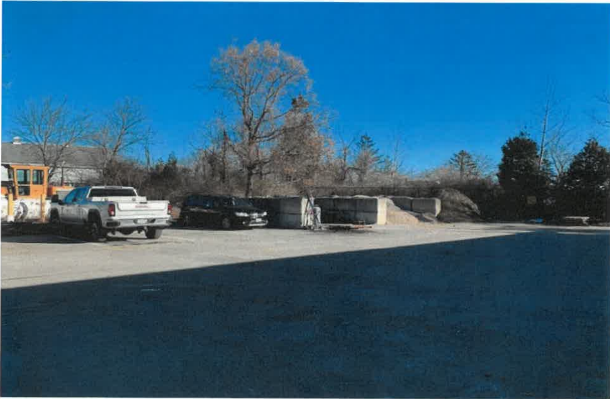
Proposed location for workshop adjacent to existing pavement in area of material bins.
