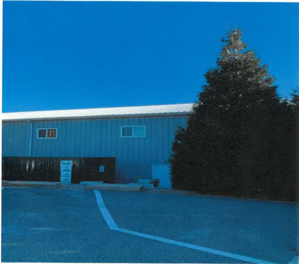
Photo taken behind police station of a building on the former CMS property. This is an example of the siding and roofing color for the proposed new workshop.
