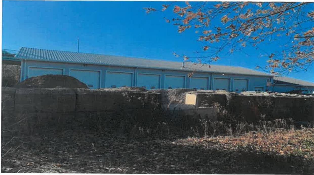
Workshop location looking south toward highway garage.
