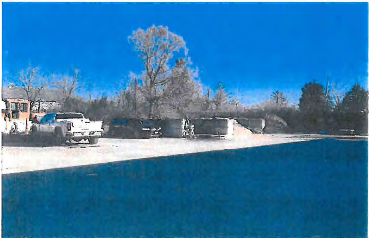
Proposed location for workshop adjacent to existing pavement in area of material bins.
