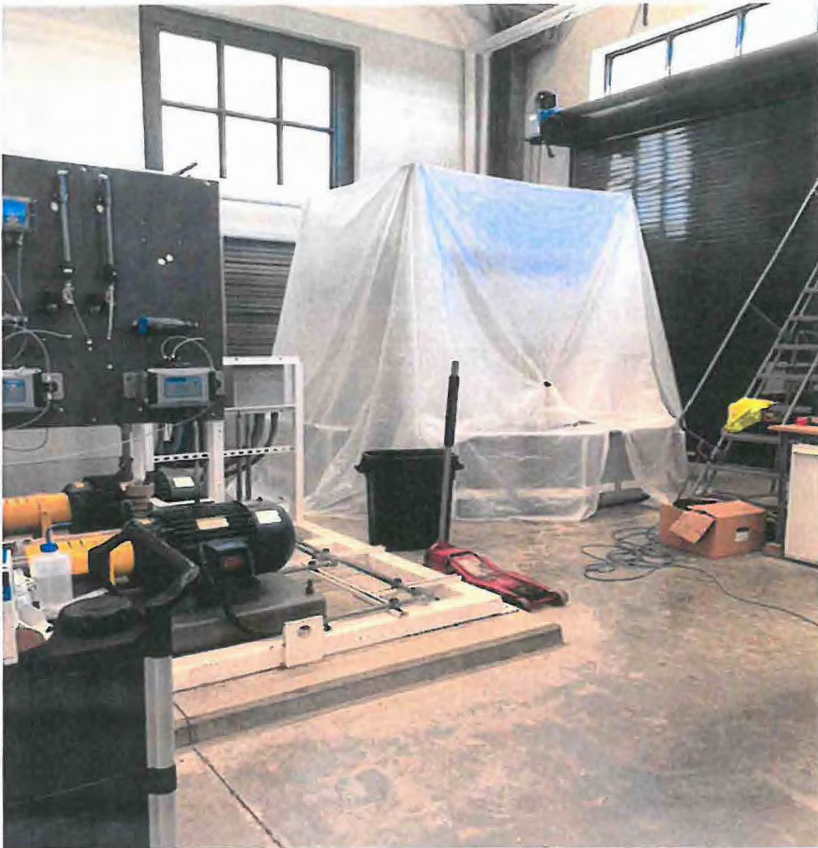
Filter for train one maintained in pool of water to keep membranes in a moist environment during tank coating
