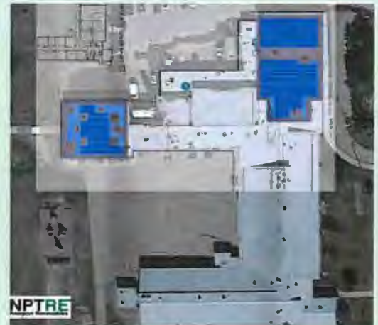
Lawn School Roof Array
