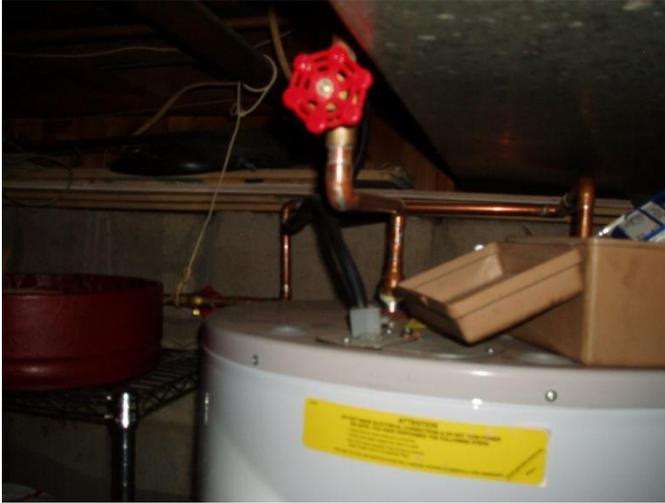
Supply wiring should be in metal conduit
