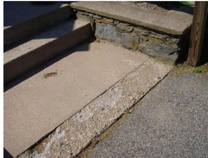
Paving corroding causing potential trip hazard
