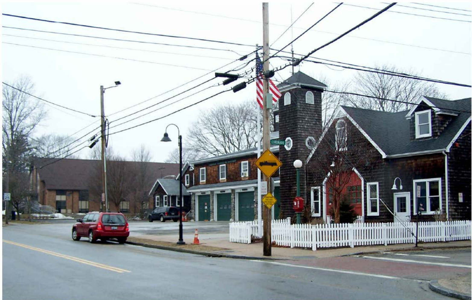
EXISTING VIEW - TRAVELING WEST ON NARRAGANSETT AVE
