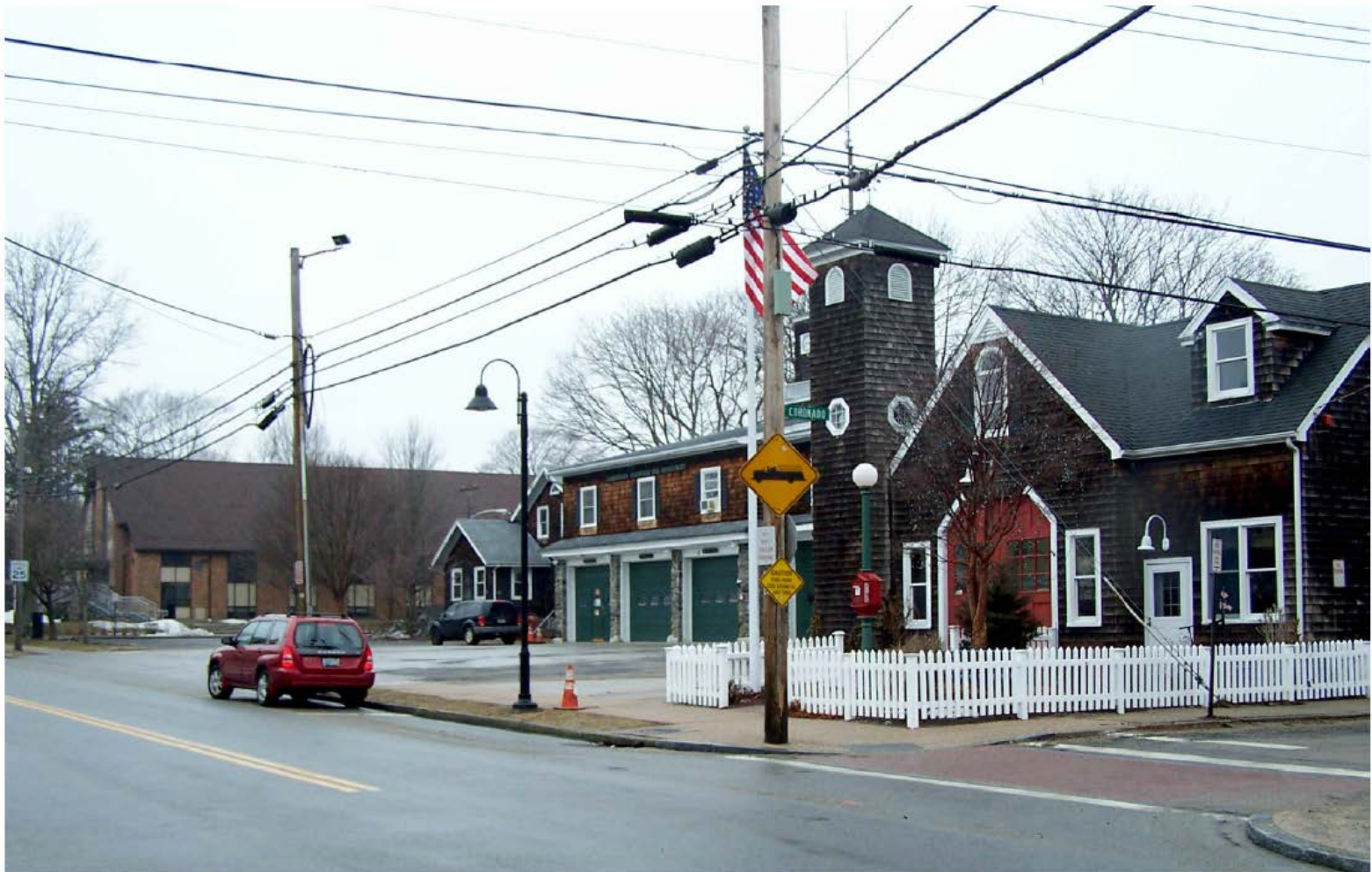
EXISTING VIEW - TRAVELING WEST ON NARRAGANSETT AVE
