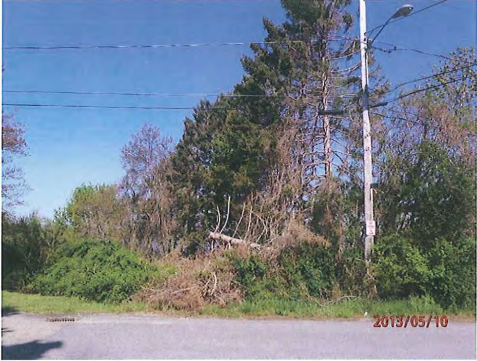
Storm Debris from Blizzard of 2013 is blocking access to path
