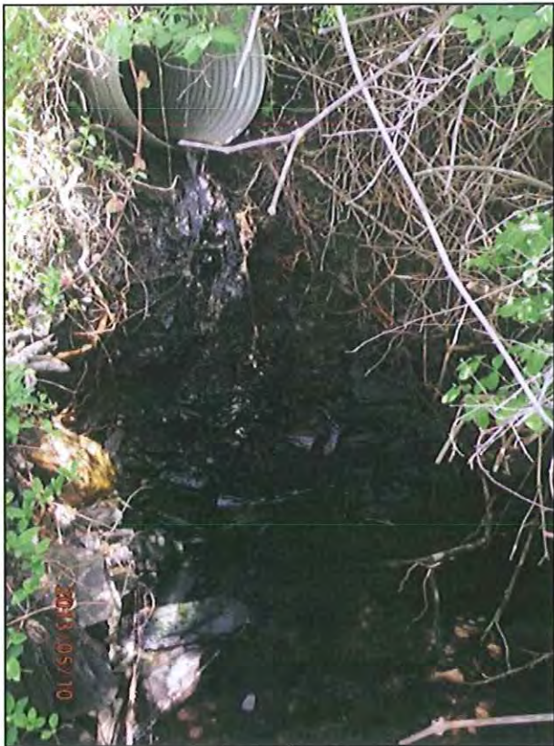
Open path maintained by abutters abruptly ends at outfall pipe and dangerous 20 foot drop. Stormwater outfall pipe is about 20 feet in from shoreline
