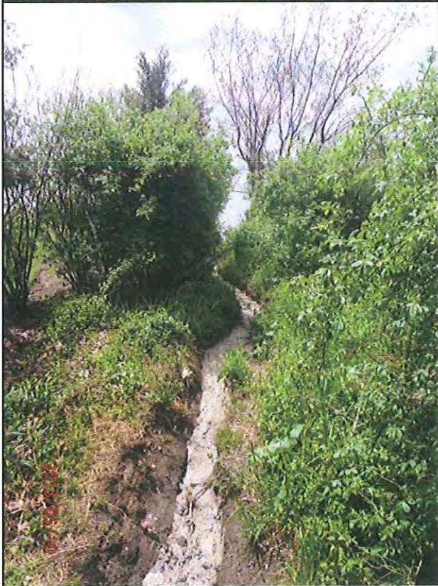
Existing footpath prone to erosion due to runoff from Capstan St
