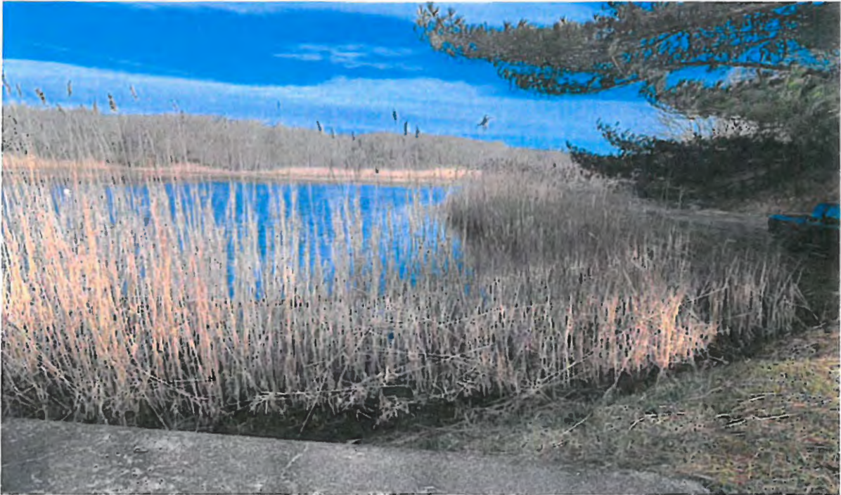
Photo looking North from the Dam spillway
