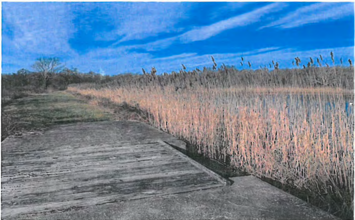
Photo looking west from Dam spillway
