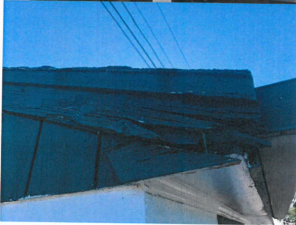
Pictured above from top left -Bottom of front door, back door, electrical panel, back window, roof
