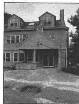
EXISTING COVERED ENTRY
