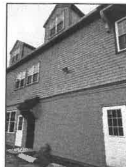
EXISTING EXTERIOR LED FLOOD LIGHTS TO REMAIN AT THREE LOCATIONS, TWO LIGHTS EAST ELEVATION, ONE LIGHT SOUTH ELEVATION
