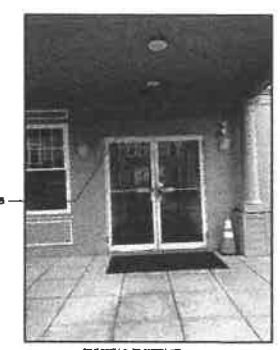
EXISTING COVERED ENTRY
