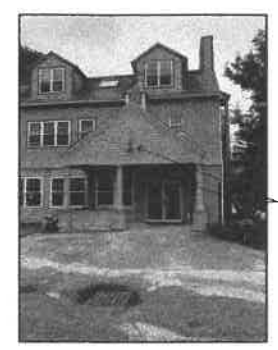
EXISTING COVERED ENTRY
