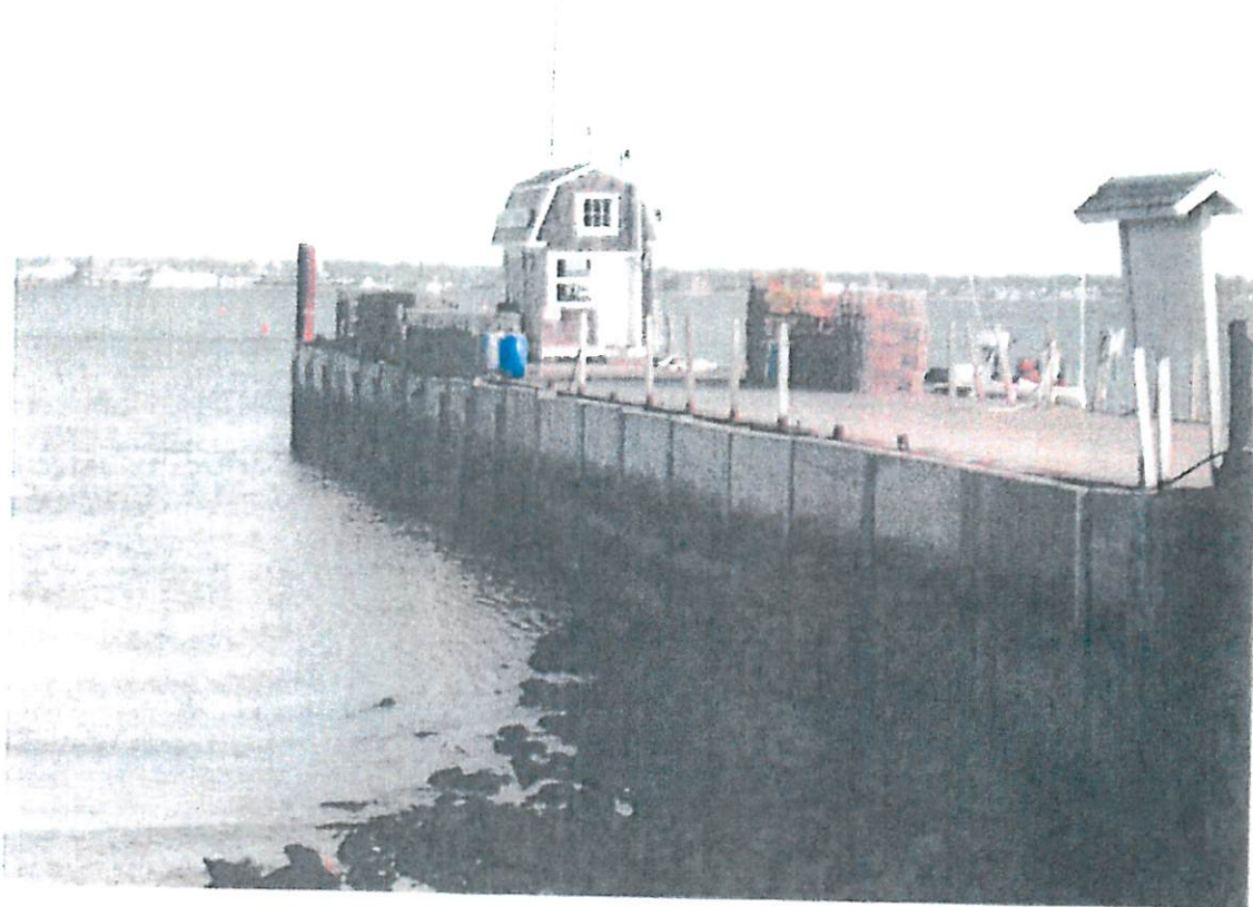
Steel Pier, Looking South, Photo Taken by RTG on January 20, 2006
