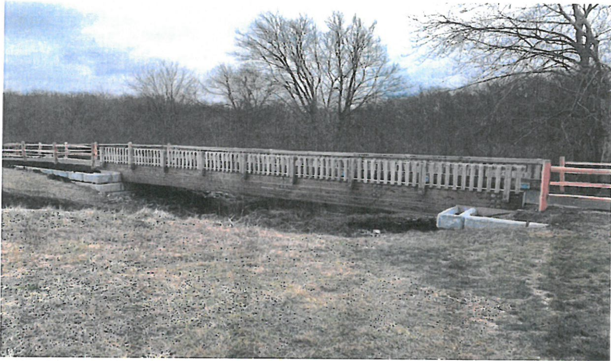
Bridge over the spillway at the Dam
