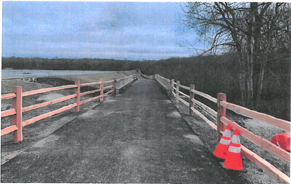
Path at entrance from North Main Road.
