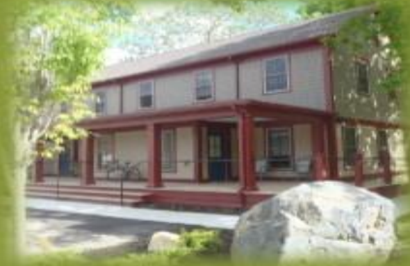
Bridges Inc. Hammett Court Apartments Union Studio Architecture
