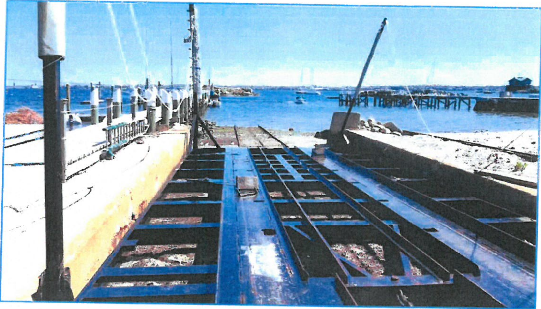
Photograph 3 – Existing marine railway looking east
