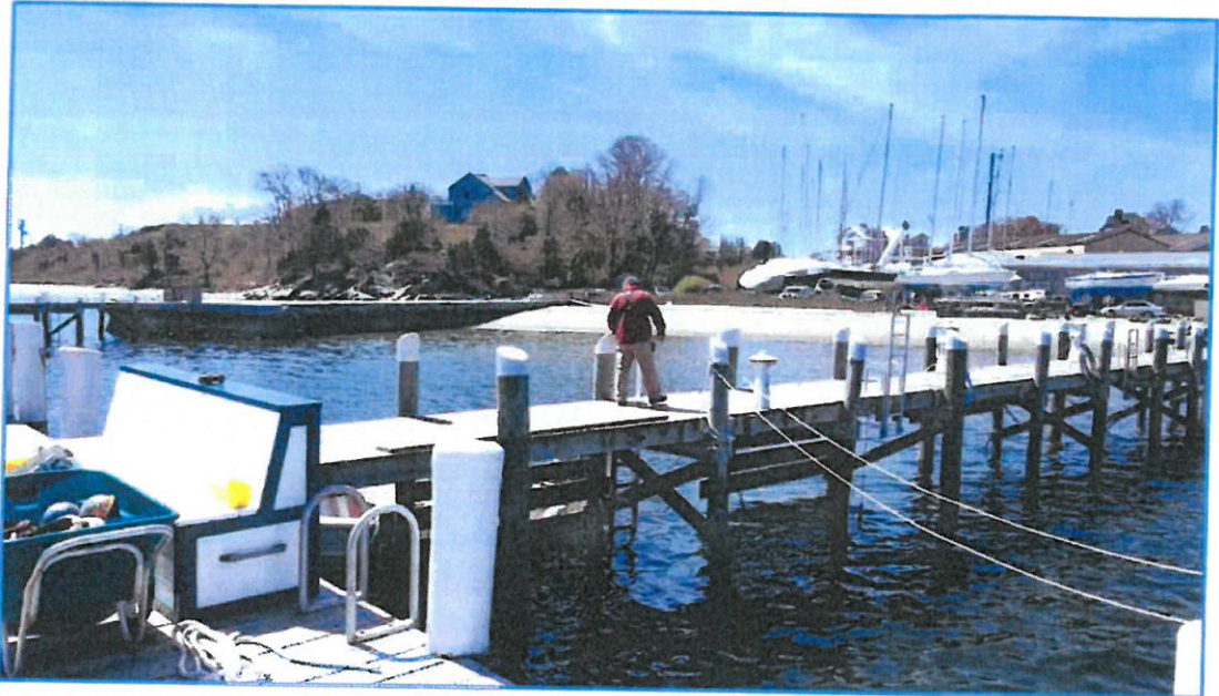
Photograph 4 – Existing site looking southwest
