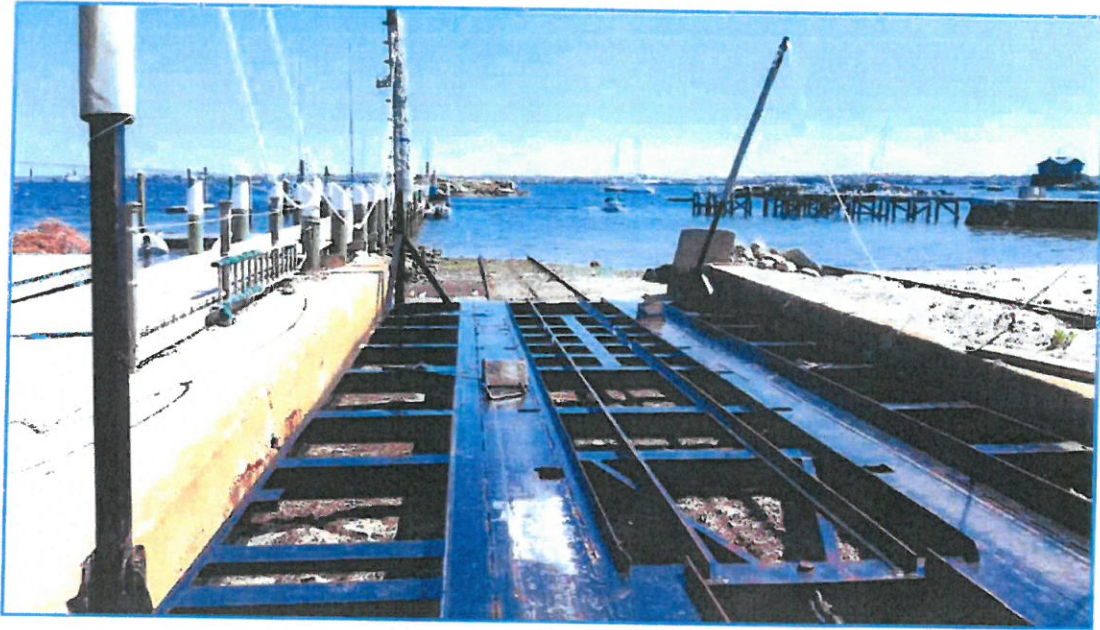
Photograph 3 – Existing marine railway looking east
