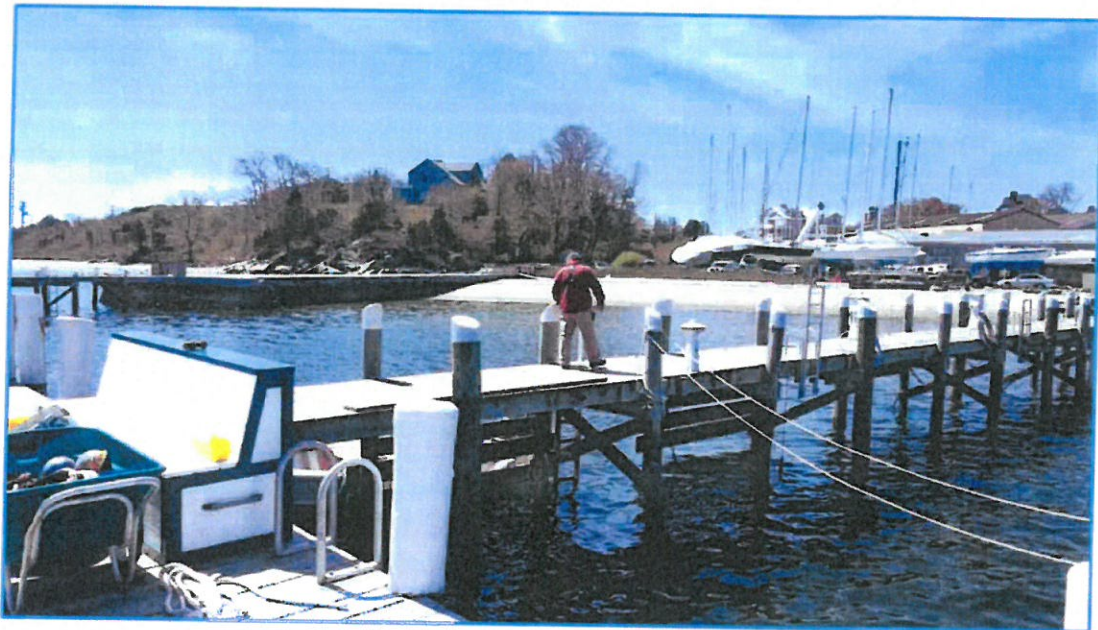
Photograph 4 – Existing site looking southwest
