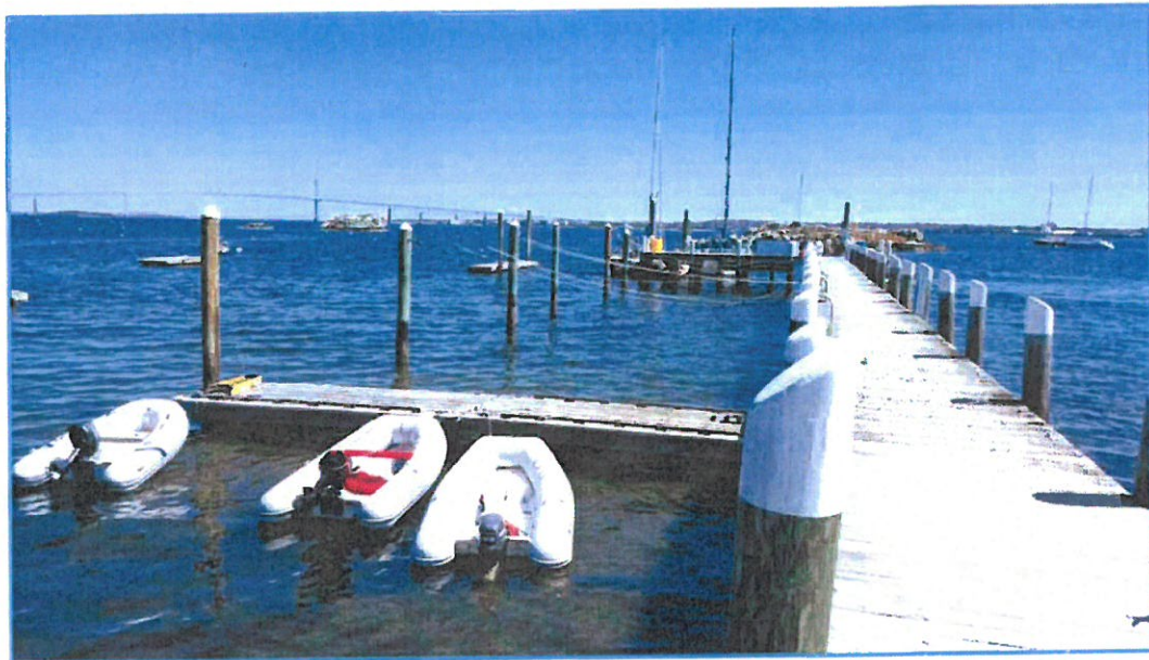
Photograph 6 – Existing pier and float looking west
