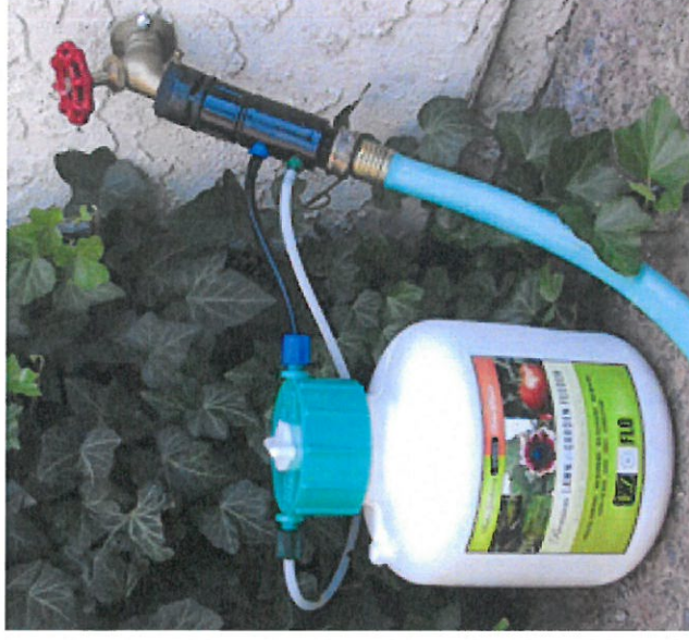
The most common Cross-Connection is a garden hose.
