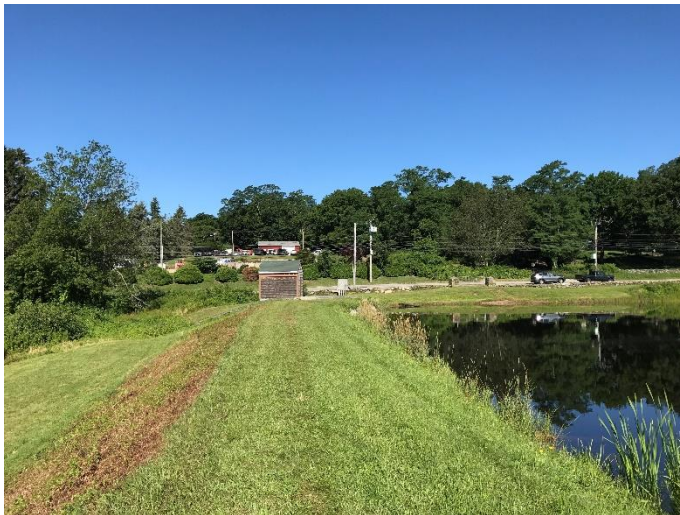
North Pond Dam – Looking West
