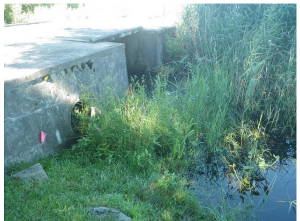
South Pond Spillway
