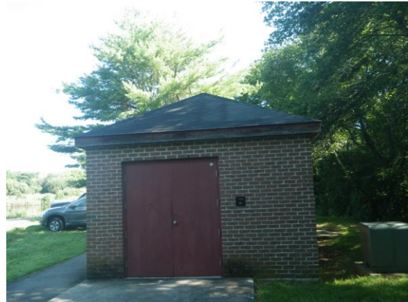
Pretreatment building at South Pond
