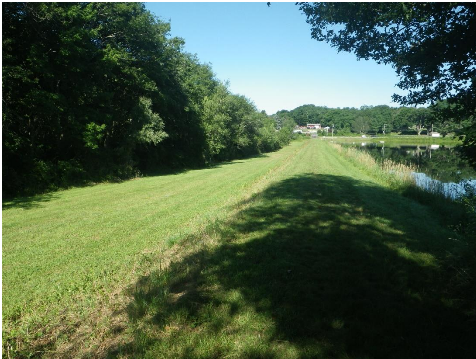
LOOKING EAST ALONG TOP OF DAM NEAR WELL JR-1
