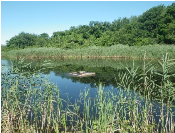
South Pond Intake Structure
