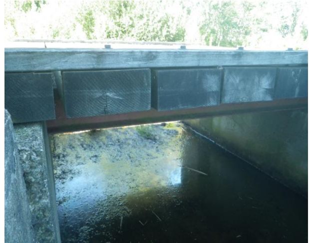
South Pond Spillway
