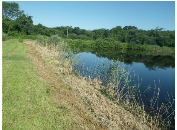
South Pond Dam Embankment
