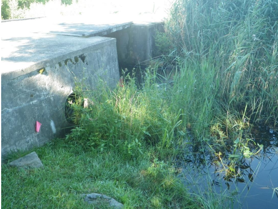
UPSTREAM SIDE OF SPILLWAY
