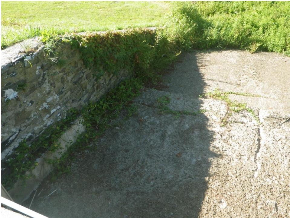
SPILLWAY ABUTMENT WALL
