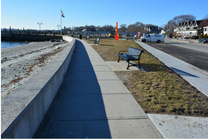
C. lawn near bus shelter
