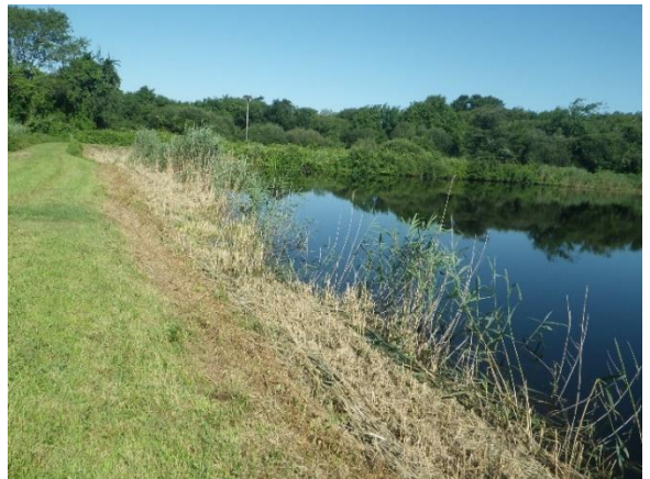
South Pond Dam Embankment
