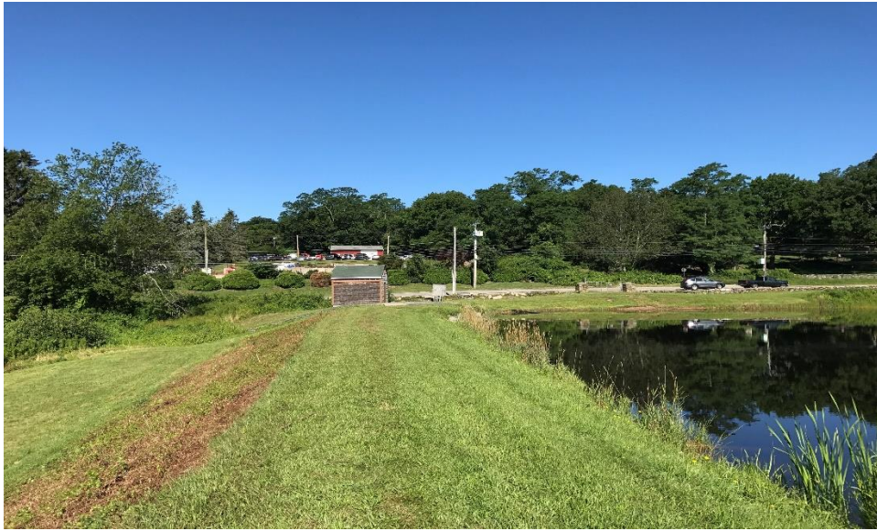
LOOKING WEST ALONG TOP OF DAM
