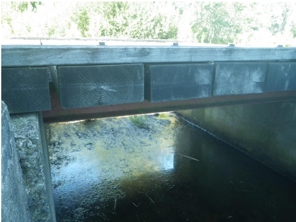
DOWNSTREAM AT SPILLWAY
