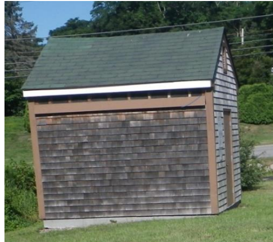
North Pond – Blower Building
