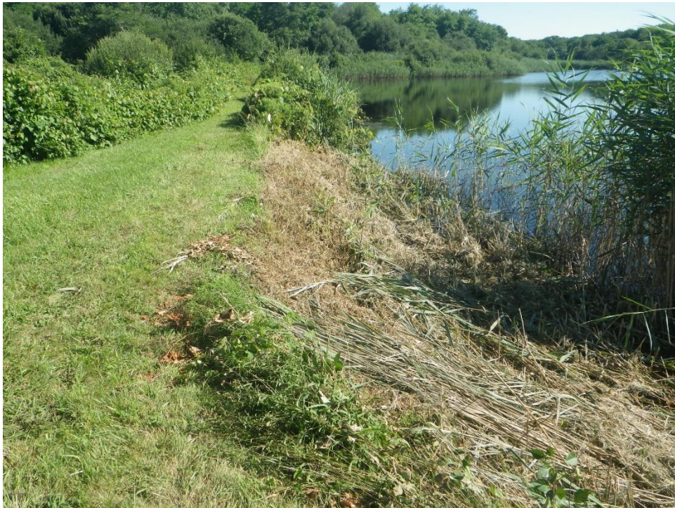
SOUTHWEST CORNER OF DIKE – LOOKING NORTH
