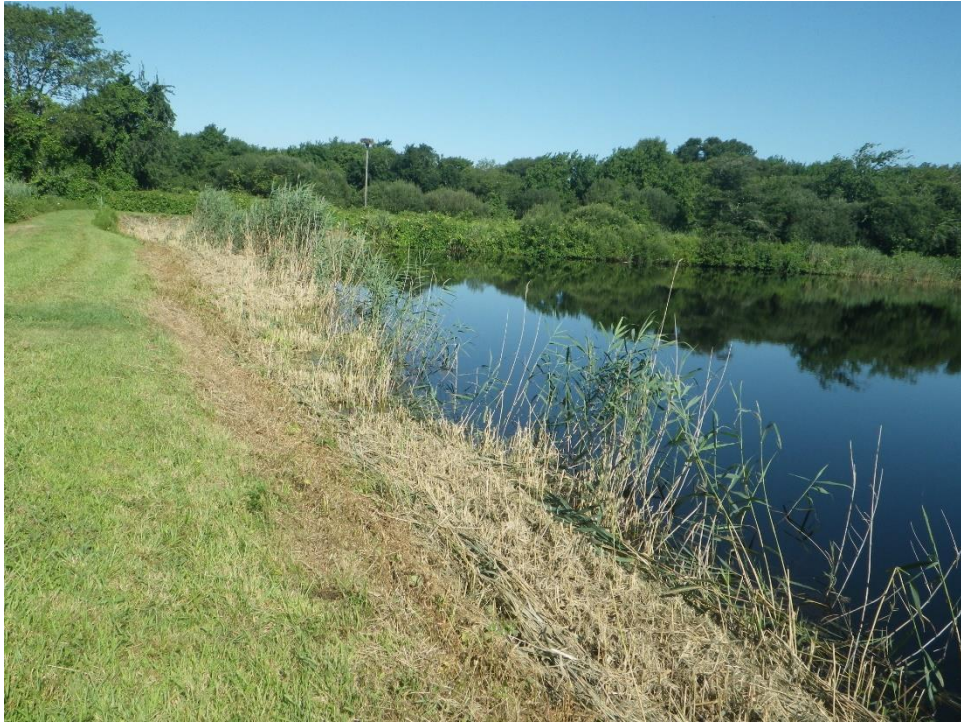
SOUTHEAST CORNER OF DAM – LOOKING WEST
