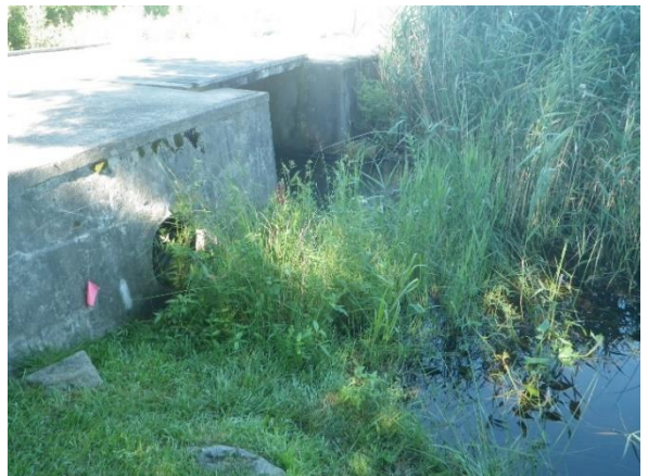
South Pond Spillway
