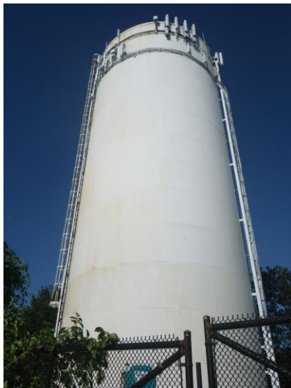
Howland Avenue Standpipe #1
