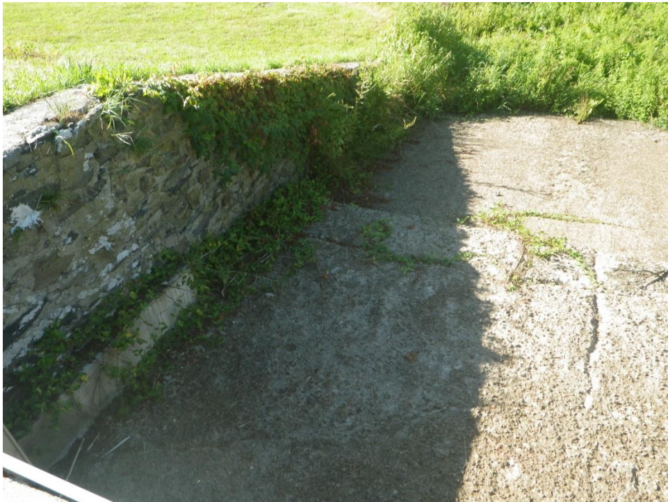
SPILLWAY ABUTMENT WALL
