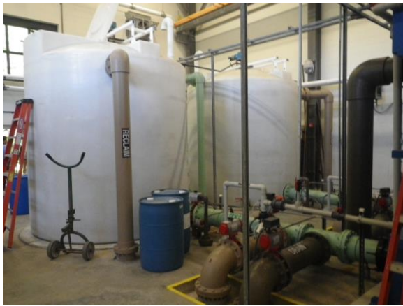
Coagulation Tanks
