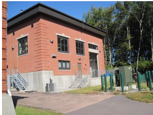
New Treatment Plant
