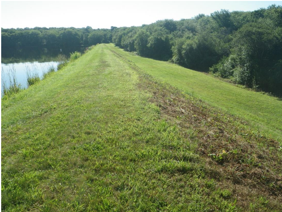
LOOKING EAST ALONG TOP OF DAM
