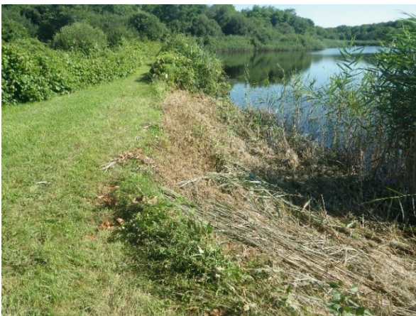
South Pond Dike Earthen Berm
