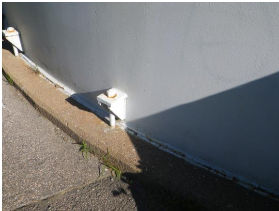
Standpipe #1 Anchor Bolts
