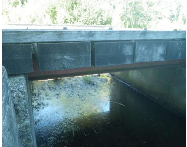
South Pond Spillway
