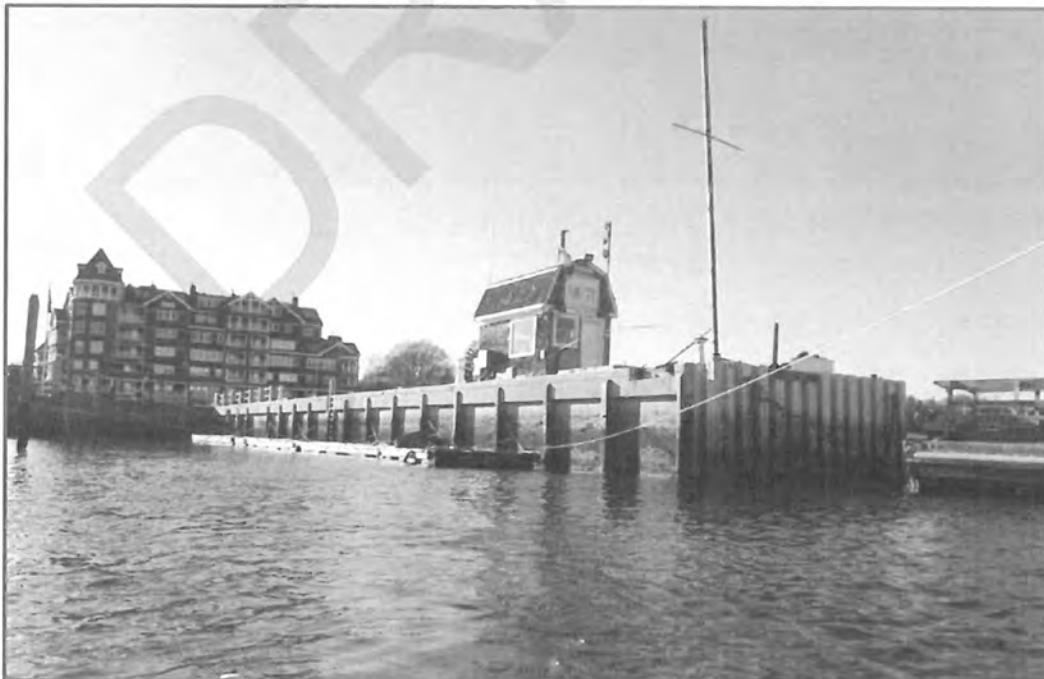
Photo No. 2: East Ferry Marina Pier, looking northwest, photo taken on March 23, 2019.
