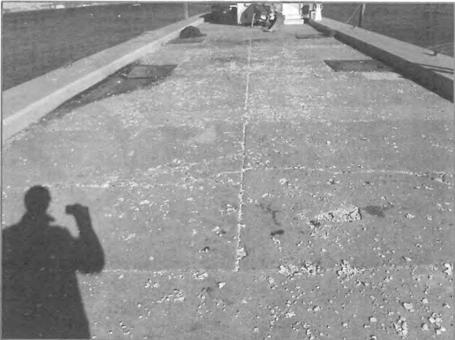
Photo No. 8: Concrete Pier Deck, looking east, photo taken on March 23, 2019.
