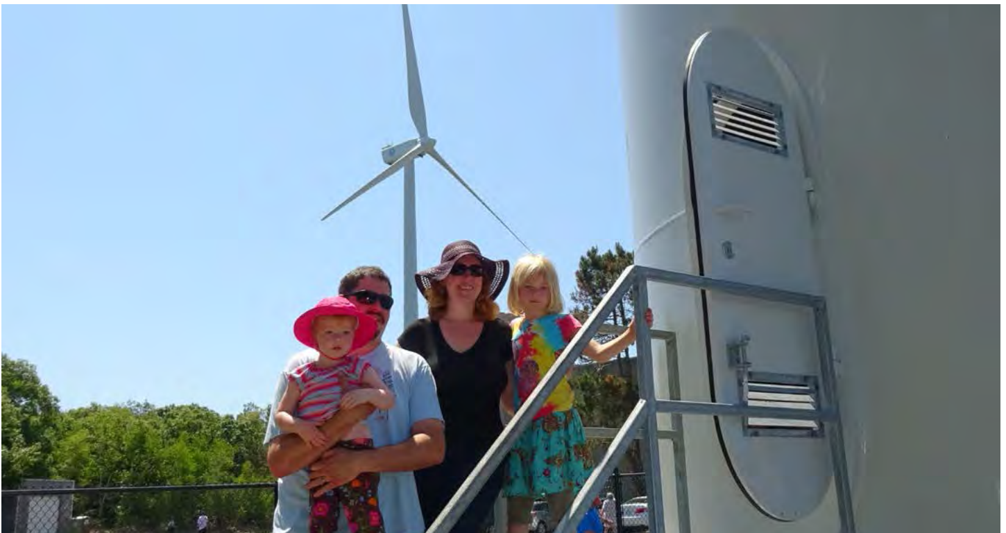
Wind turbines in Gloucester, MA
