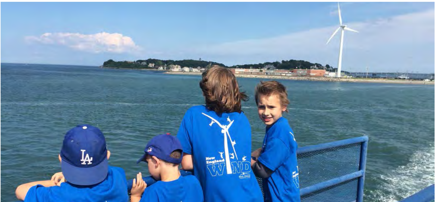
Hull 1 Wind Turbine
