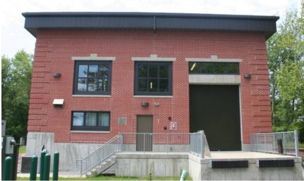
The Jamestown Public Water Supply system has a pre-treatment facility at South Pond. This facility was designed to provide chemical treatment for disinfection, taste, and odor control, color reduction, pH adjustment, and flow monitoring. This facility has the capability to treat up to 500,000 gallons per day with the existing chemical feed pumps.
