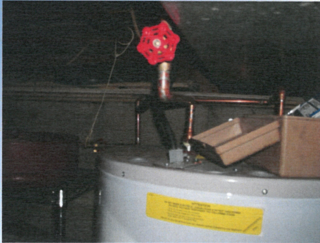
Supply wiring should be in metal conduit
