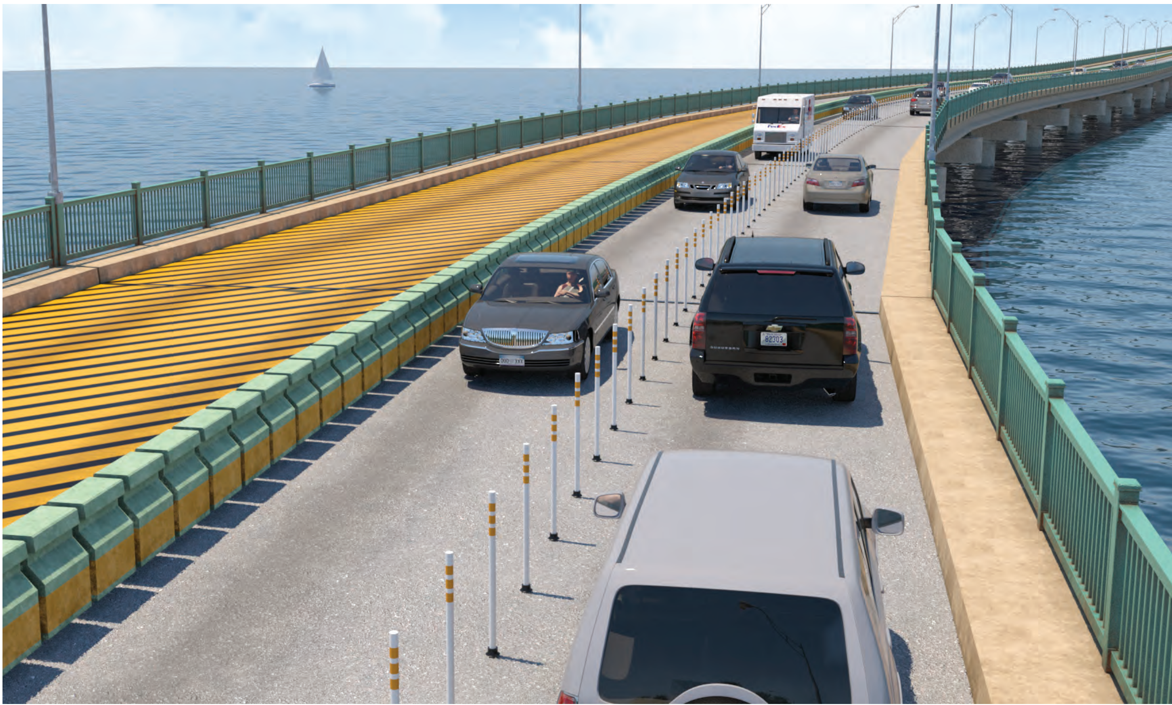
Traffic pattern implemented on the Newport Pell Bridge during lane closure periods.
