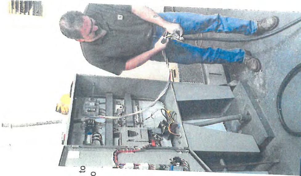
Top: Superintendent Ouellette wires a RAS pump. Right: Our new Sewer Jet with camera option.
