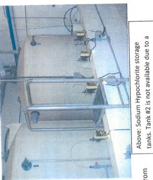
One of our Sodium Hypochlorite tanks has a leak. As a result we cannot use it. We are researching ways to either repair the tank or replace it.
