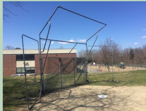
Location of soon to be constructed new backstop
