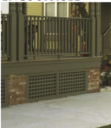
25.2 Infill panels between porch foundation piers are often lattice.
