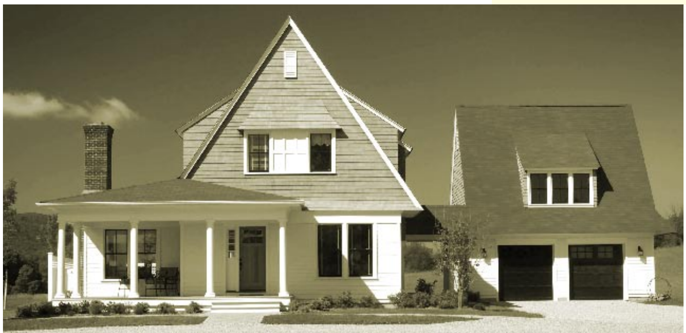
11.4 The garage is deferential to the main house by having a lower roof spring line than that of the main house. However, the two structures share similar materials and proportions, creating an aesthetic harmony among all parts.
