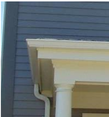
19.2 Ogee gutters should return with the eave or entablature and die into the face of the house.
