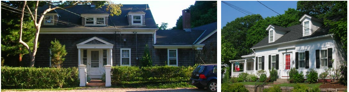
10.2 A backbuilding connects the main house with an addition. There is a hierarchy among the three pieces that can be understood from the scale of each.
