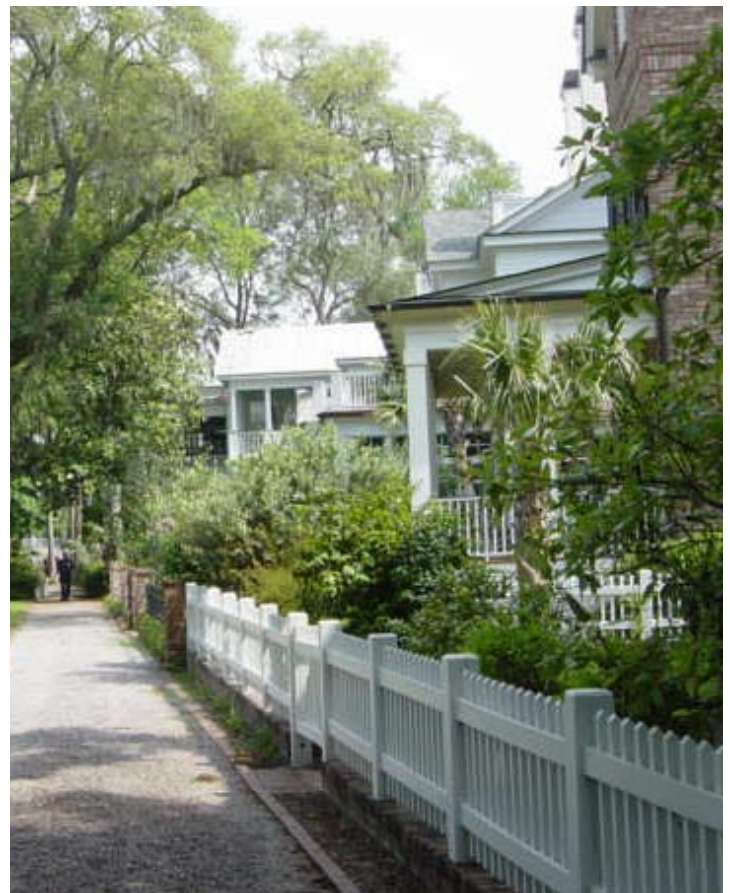
30.2 A picket fence set on a brick foundation protects it from ground water and rot. The combination of fences and landscaping along this sidewalk creates a strong line between the public realm and private property.
