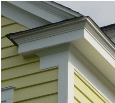
18.2 Encouraged. Appropriate eave return at a gable end. Flashing / waterproofing on top surface of gable return is not visible when viewing the façade - and in no case should be greater than 1:12. The primary eave trim and detailing is carried fully around - symmetrically disposed about the corner board.
