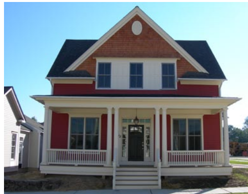
6.3 Generally, a single dominant roof form is clearly legible, with the roofs of secondary masses deferring in scale to the main body of the building.
