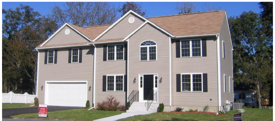
6.5 This building has a very simple massing that has been overly complicated by too many roof forms.
