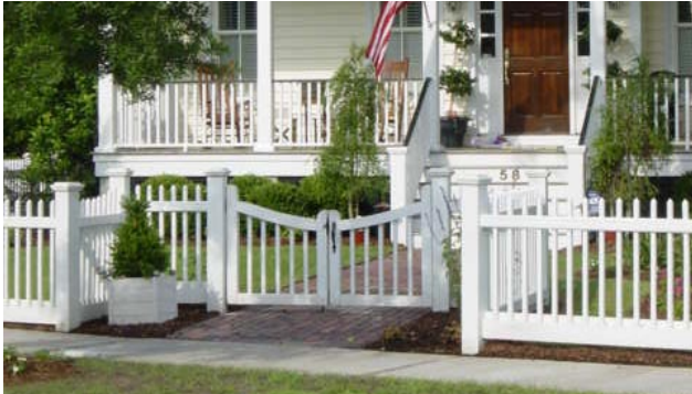
30.2 An inset gate marks the entry to the house.
