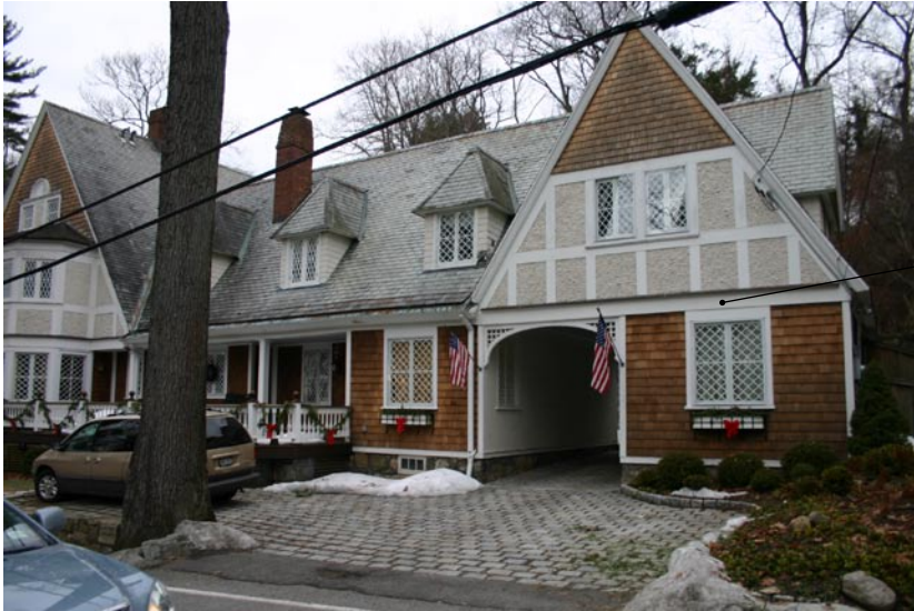
16.1 Changes in material occur here to emphasize specific building volumes. Despite the use of several materials, there is a harmony among the parts.
