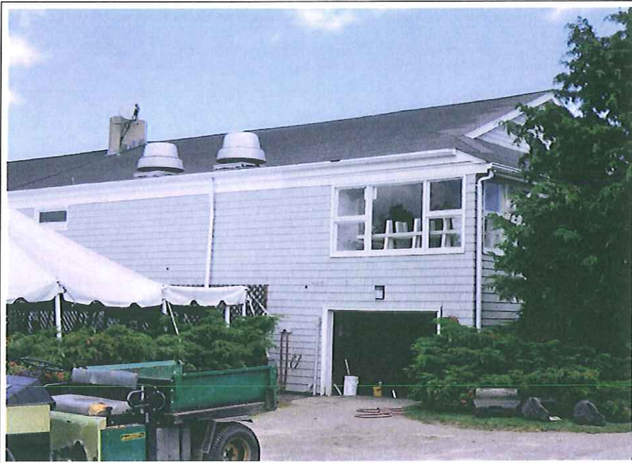
Photo 1 Southwest corner of Jamestown Golf Course building.
