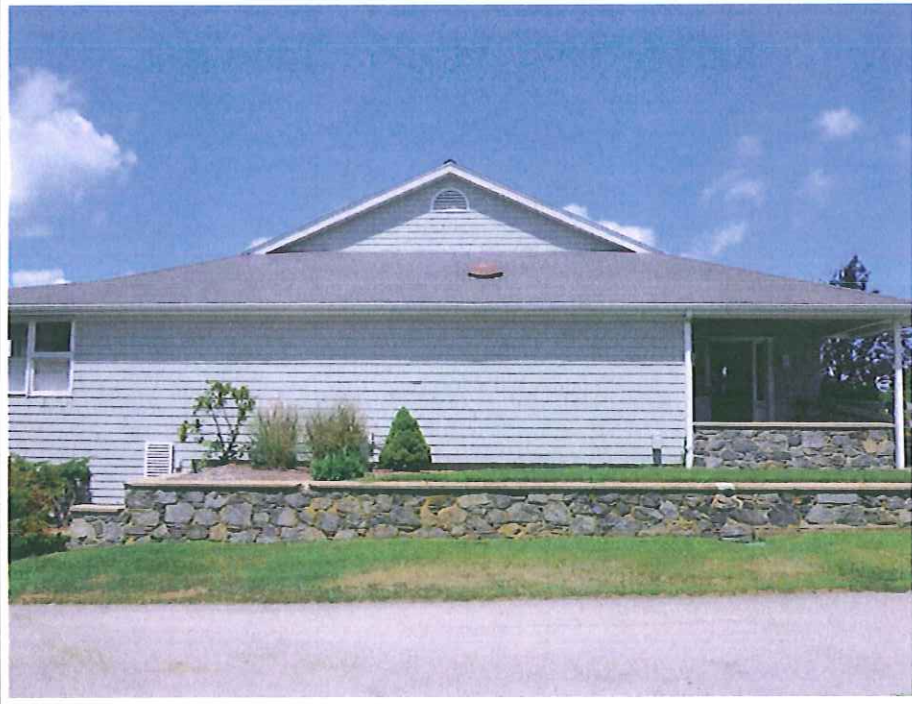
Photo 2 South elevation of Jamestown Golf Course building.
