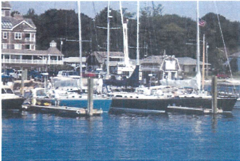
The CMS dock office overlooking sailboats in the marina.
