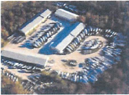
Taylor Point storage and repair site. Photo: Onne Van der Waal.
