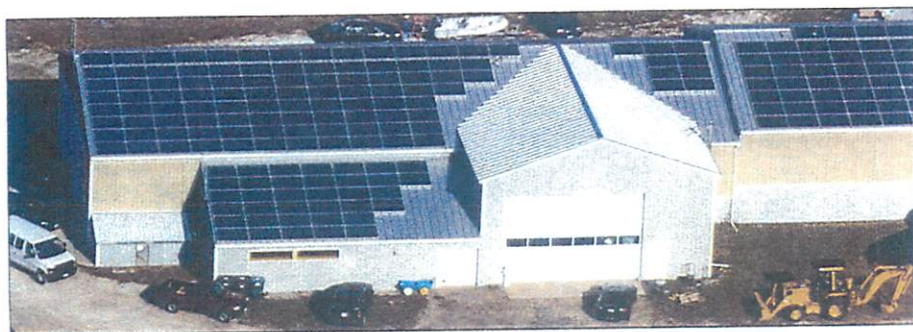
The full 100kW system at Kingman Yacht Center in Cataumet, Cape Cod, Massachusetts spans three roofs
