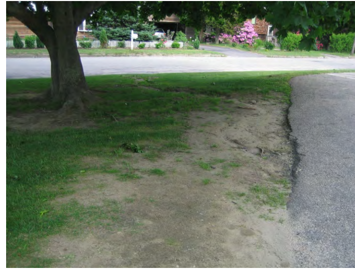
Lack of Curbing: Vehicular compaction has damaged grass and lead to increased erosion
