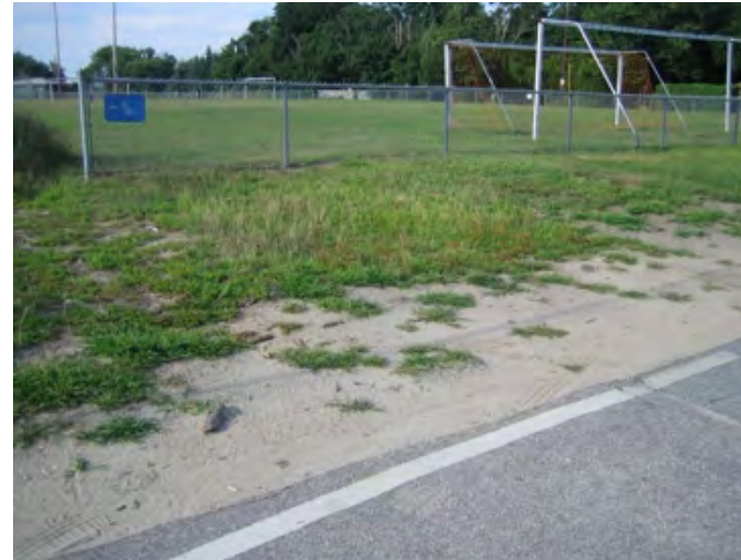
Erosion at edge of pavement due to overflow parking adjacent to Lawn Avenue School
