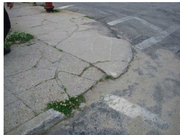
Deteriorating Wheel Chair Ramp
