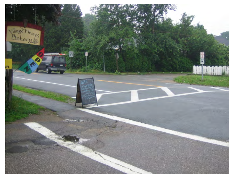
Crosswalk at North Road and Watson Ave. (Pavement inadequate, sign obstructs pedestrian crossing, no sidewalk on the east side.)
