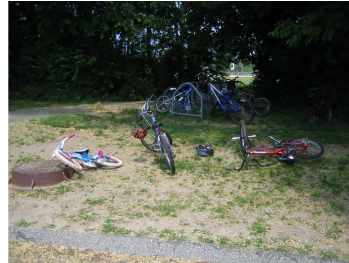
Bike storage area: Inadequate surfacing in high traffic area leads to soil erosion.
