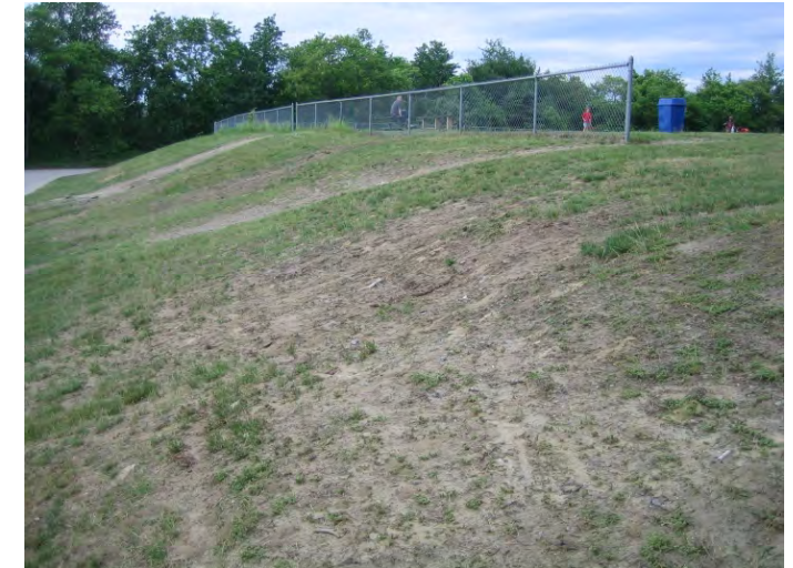
Poor soils result in inadequate slope stabilization and poor grass establishment
