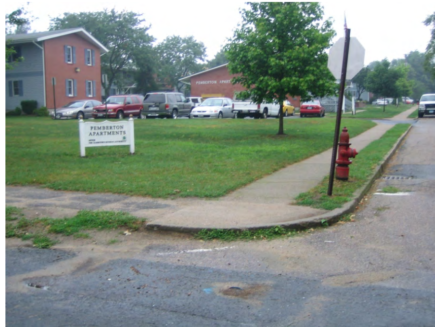
Intersection of Watson Ave. and Pemberton Ave. - west side (No handicap ramp and no crosswalk designation.)
