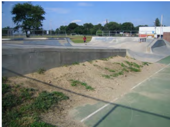
Typical Erosion at edges of skatepark
