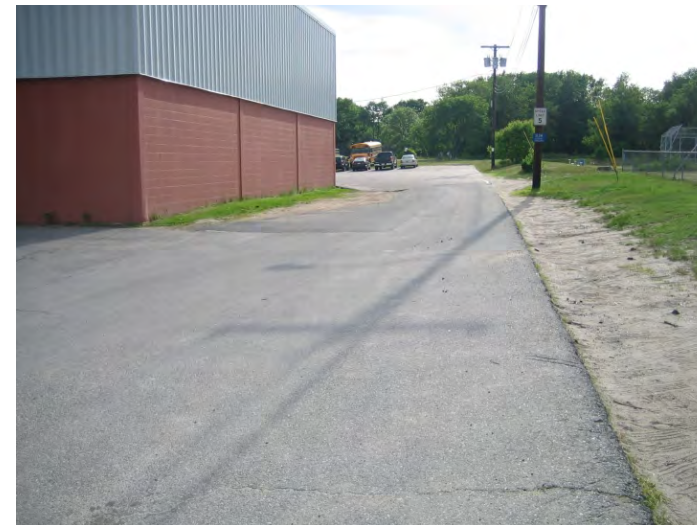
Un-Restricted parking along edge of pavement accelerates erosion
