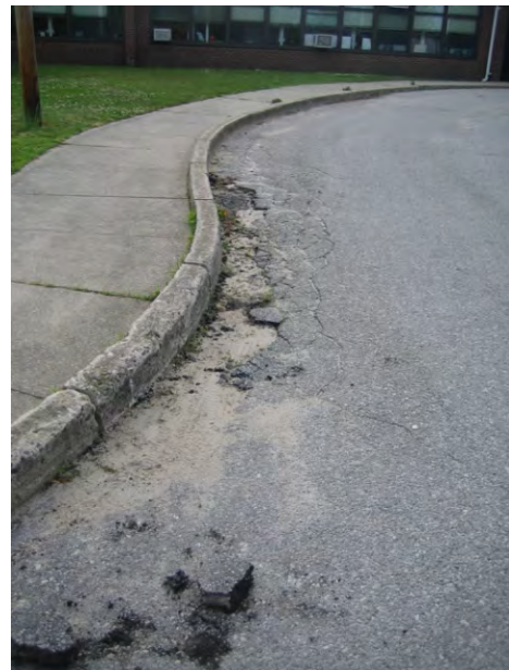
Deteriorating Asphalt and Settlement
