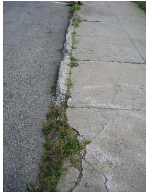
Broken Curb and broken concrete sidewalk
