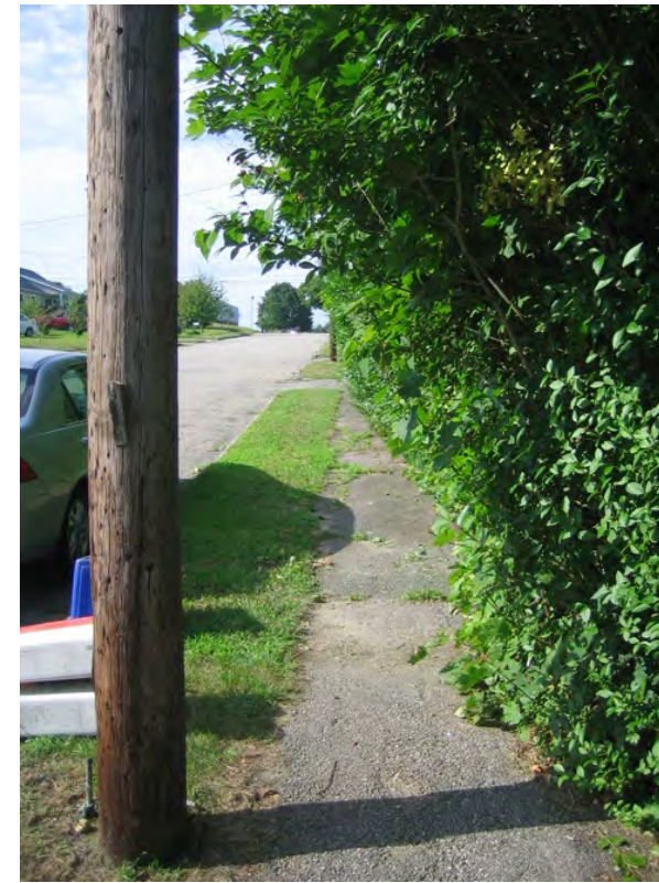
Overgrown hedges and poor pavement conditions and a utility pole make this section of sidewalk difficult to traverse
