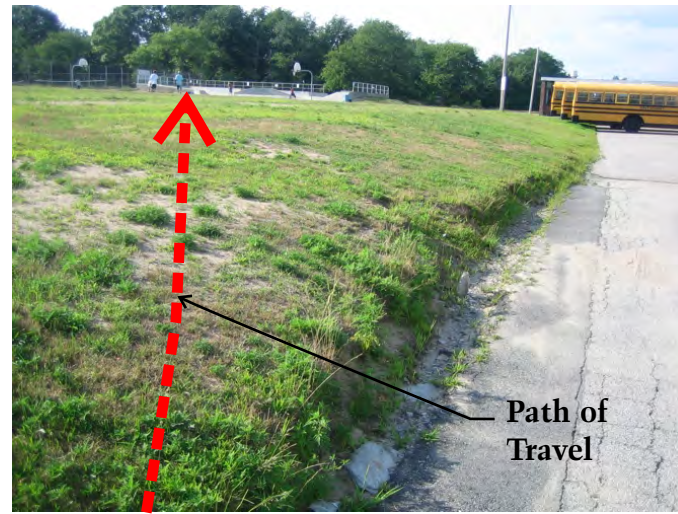
Desire line from Watson Avenue to skatepark (note severe erosion at the edge of pavement)
