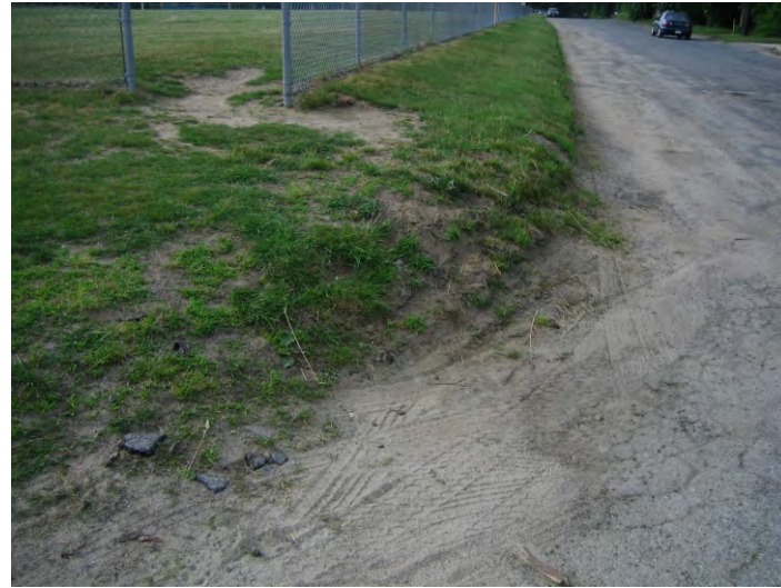
Overland drainage across gravel shoulder caused sedimentation problems
