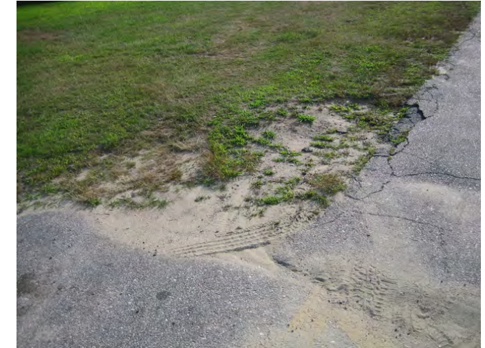
Inadequate pavement width where path leads to erosion
