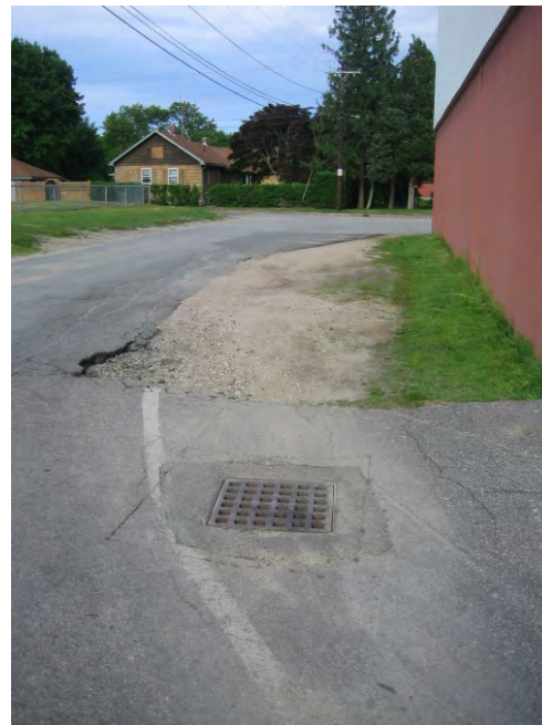
Road edge disturbance due to heavy traffic and bus circulation
