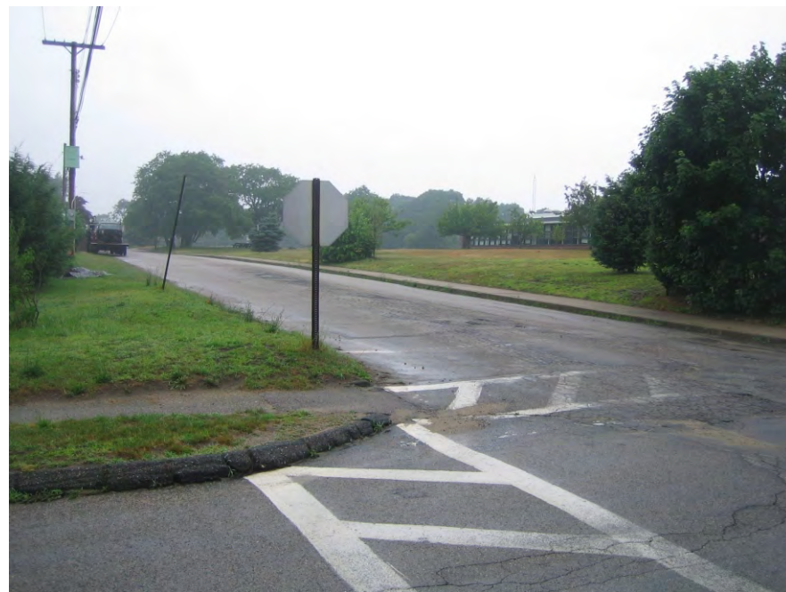
Watson Avenue & Lawn Avenue (Irregular road surface, broken curbing, vegetation encroachment and deteriorating crosswalk striping)
