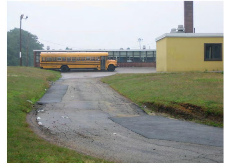
Inadequate Pavement: Narrow driveway width forces traffic to edges of pavement
