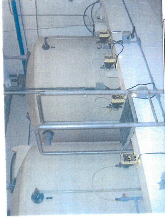
Above: Sodium Hypochlorite storage tanks. Tank #2 is not available due to a leak.
