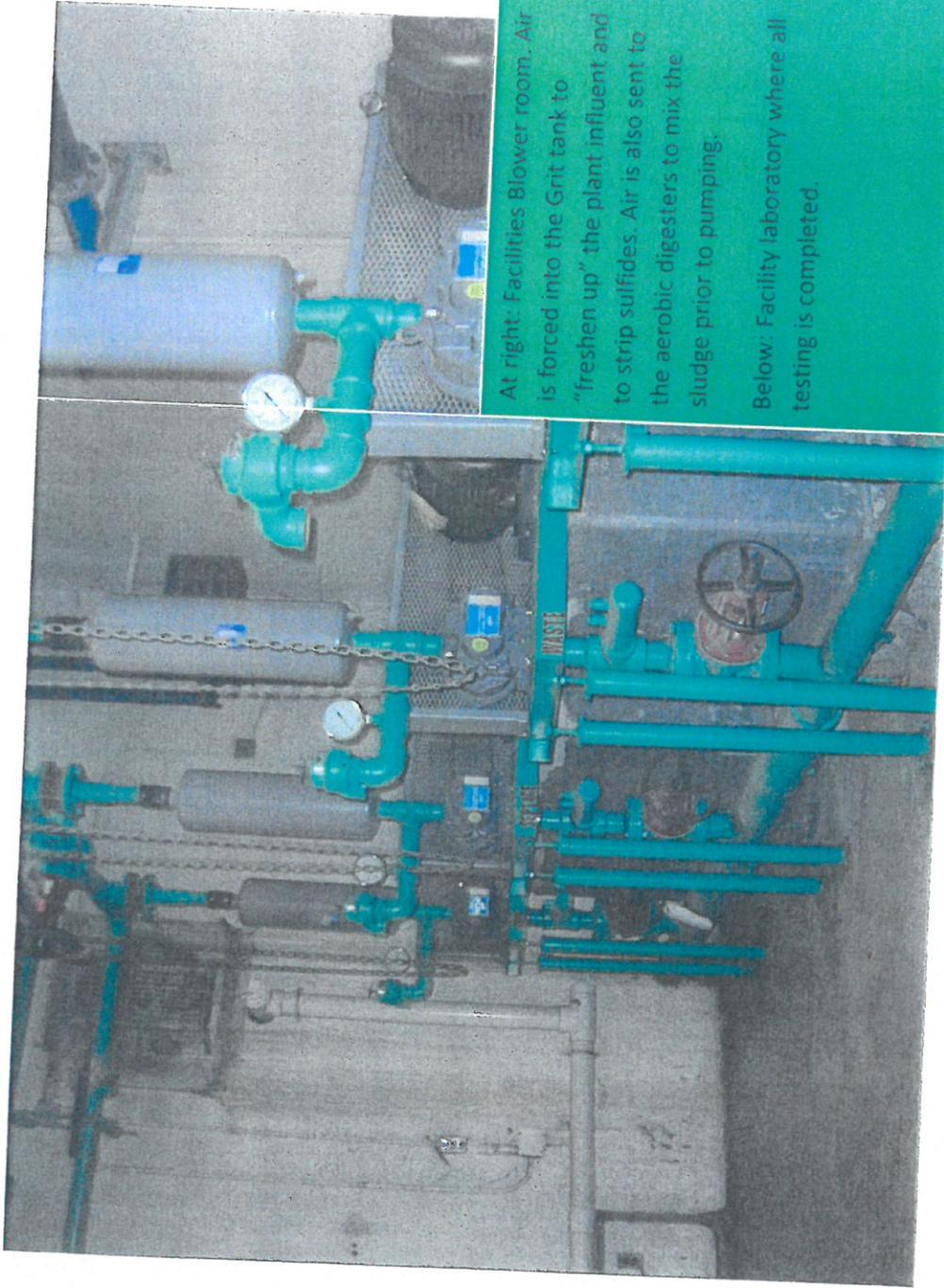
At right: Facilities Blower room. Air is forced into the Grit tank to "freshen up" the plant influent and to strip sulfides. Air is also sent to the aerobic digesters to mix the sludge prior to pumping.
