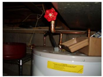
Supply wiring should be in metal conduit
