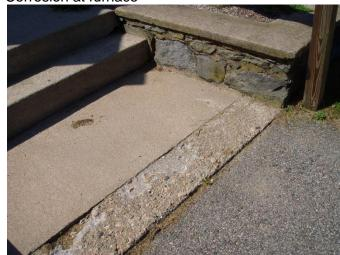
Paving corroding causing potential trip hazard
